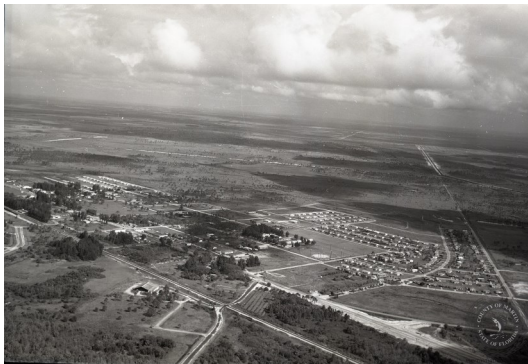
Aerial of Indiantown, c. 1960
